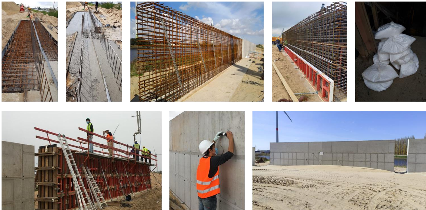
Figure 6.11 - Different stages of the testing campaign: from the casting of the slab until the monitoring of the walls.
