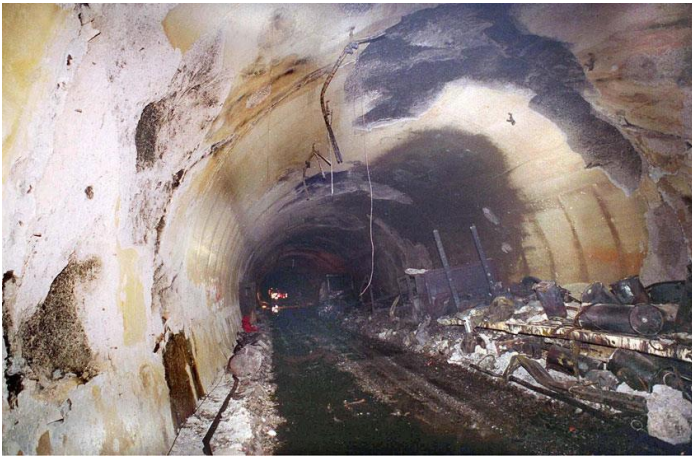
Figure 1.2 Fire damage of the tunnel lining, taken from [7].
