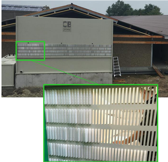
Figure 1-8: Polypropylene air-to-air heat exchanger in barn [24]
